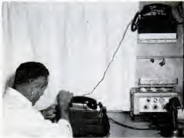
Communication section in front of trailer has two-way radio, portable phones and public-address unit
